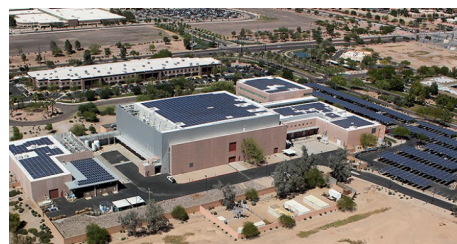
The AEP core facility is located on ASU's Science Park, a few miles from the main campus.
